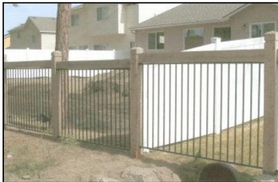
The photo above is a depiction of the fence at Ponderosa Ridge, where the wrought iron fence is required in specific areas. Please note how the fence connects into the vinyl fencing if applicable. The vinyl post connects behind the wrought iron fencing, so it is concealed from exterior of fence.
